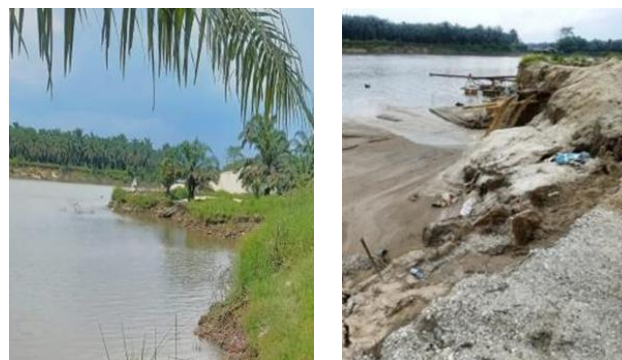
Figure 2. Erosion of the Kampar riverbank cliffs at illegal sand mining sites
